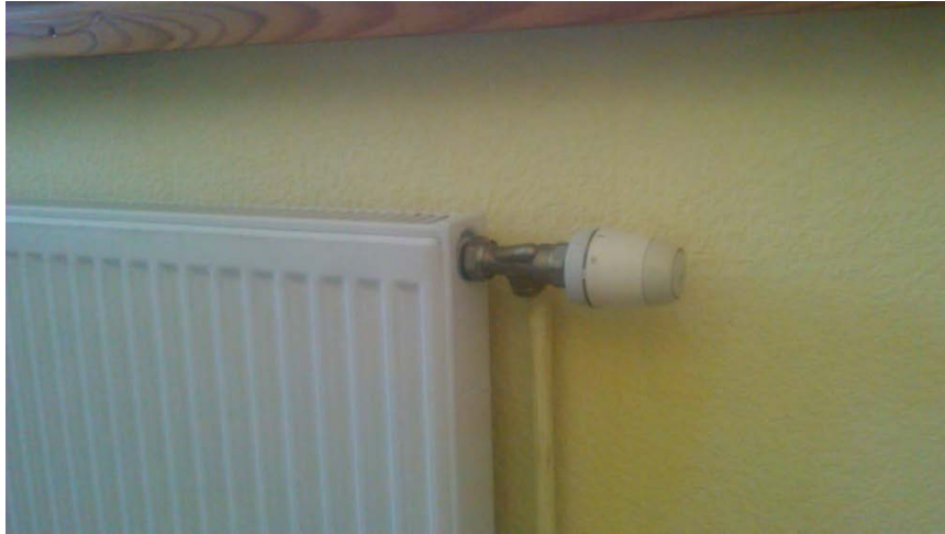
Figure 1.2. Installed radiators with thermostats
