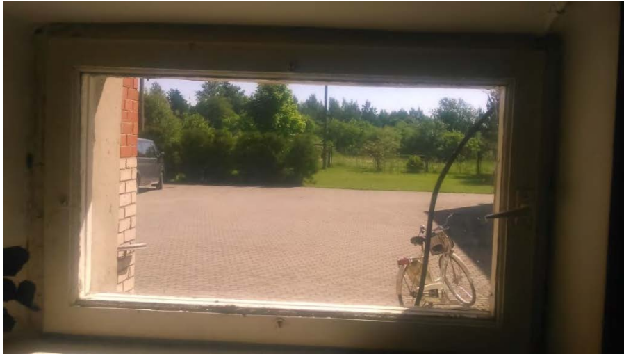
Figure 1.4. Old wooden windows without sealing
