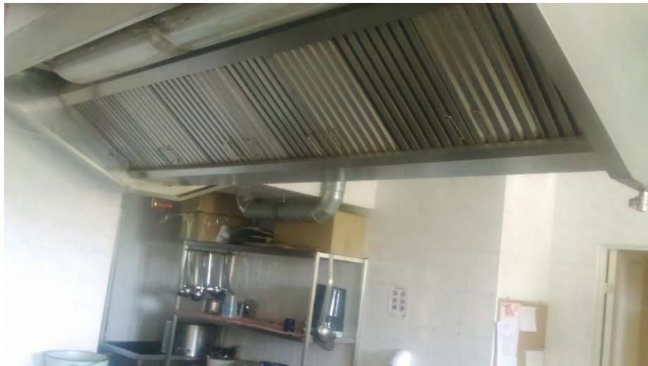
Figure 1.3. Kitchen ventilation system
