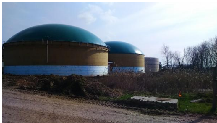
The fermentors of the biogas power plant in Harsány. Source: [18]
