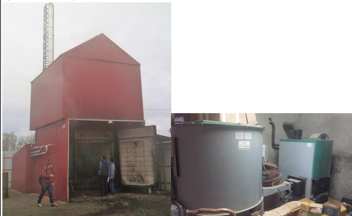
At the left: straw-fired furnace provides heat to the public buildings in Böcs. At the right: wood-chips furnace in Bükkszentkereszt (source: Adam Harmat)
