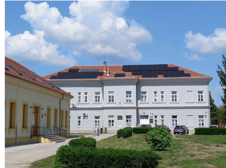
Administrative building of Medimurje County Knowledge Center complex Bana Josipa Jelačića 22 40 000 Čakovec Croatia
