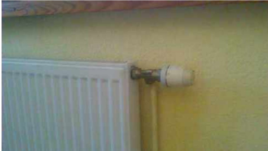
Figure 1.2. Installed radiators with thermostats
